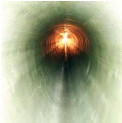
Egg-shaped section 600/900 rehabilitated with a GRP inliner
