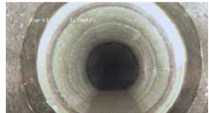
Damage rehabilitated with short liner
