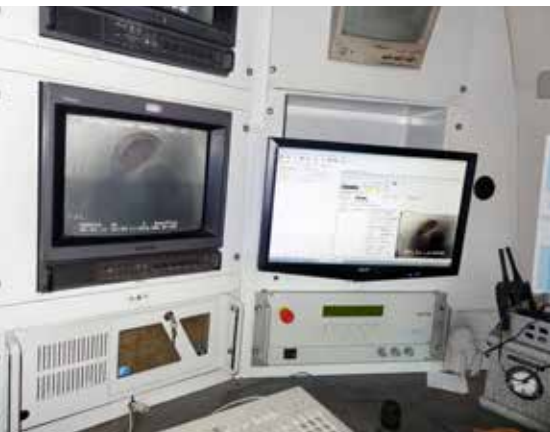
Inside view short liner plant
