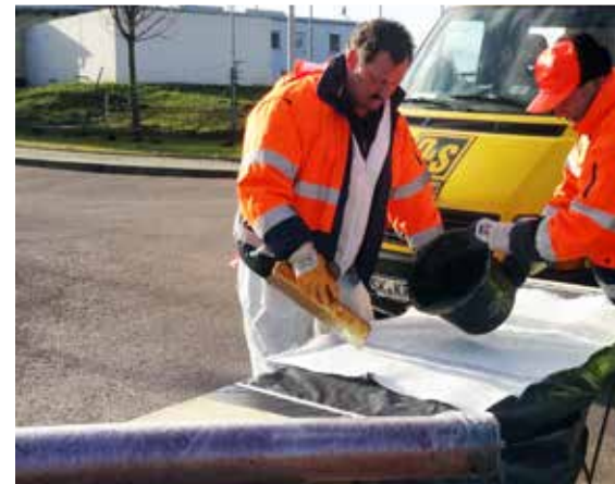
Impregnation of the short liner
