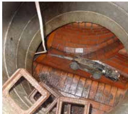
Camera monitoring short liner installation
