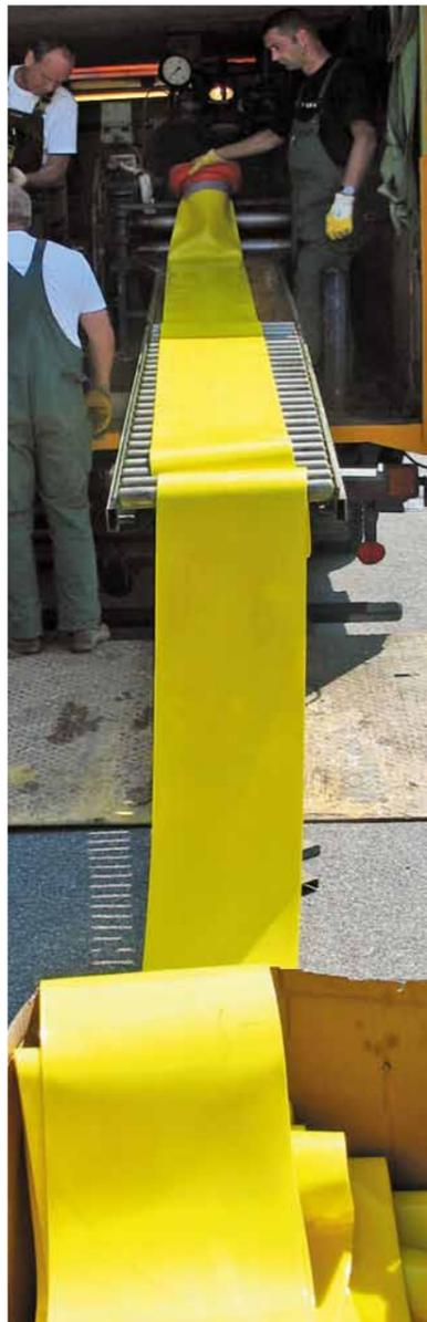
*The liner is prepared on the conveyor belt for the filling with the two-component resin*
