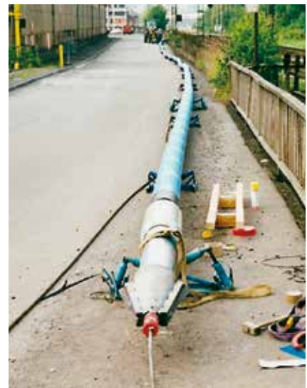
Pipe run with cutter head
