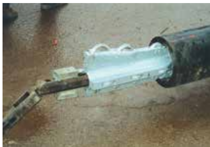
Rotary cutter for a static burst lining
