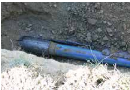
Bursting head with PE pipe run
