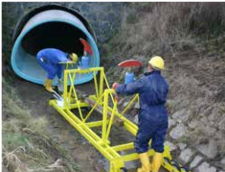
Positioning of the pipe carriage for receiving the relining section
