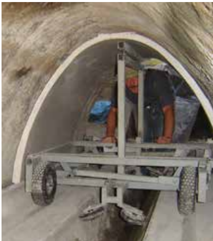
Installing the modules with the aid of a carriage
