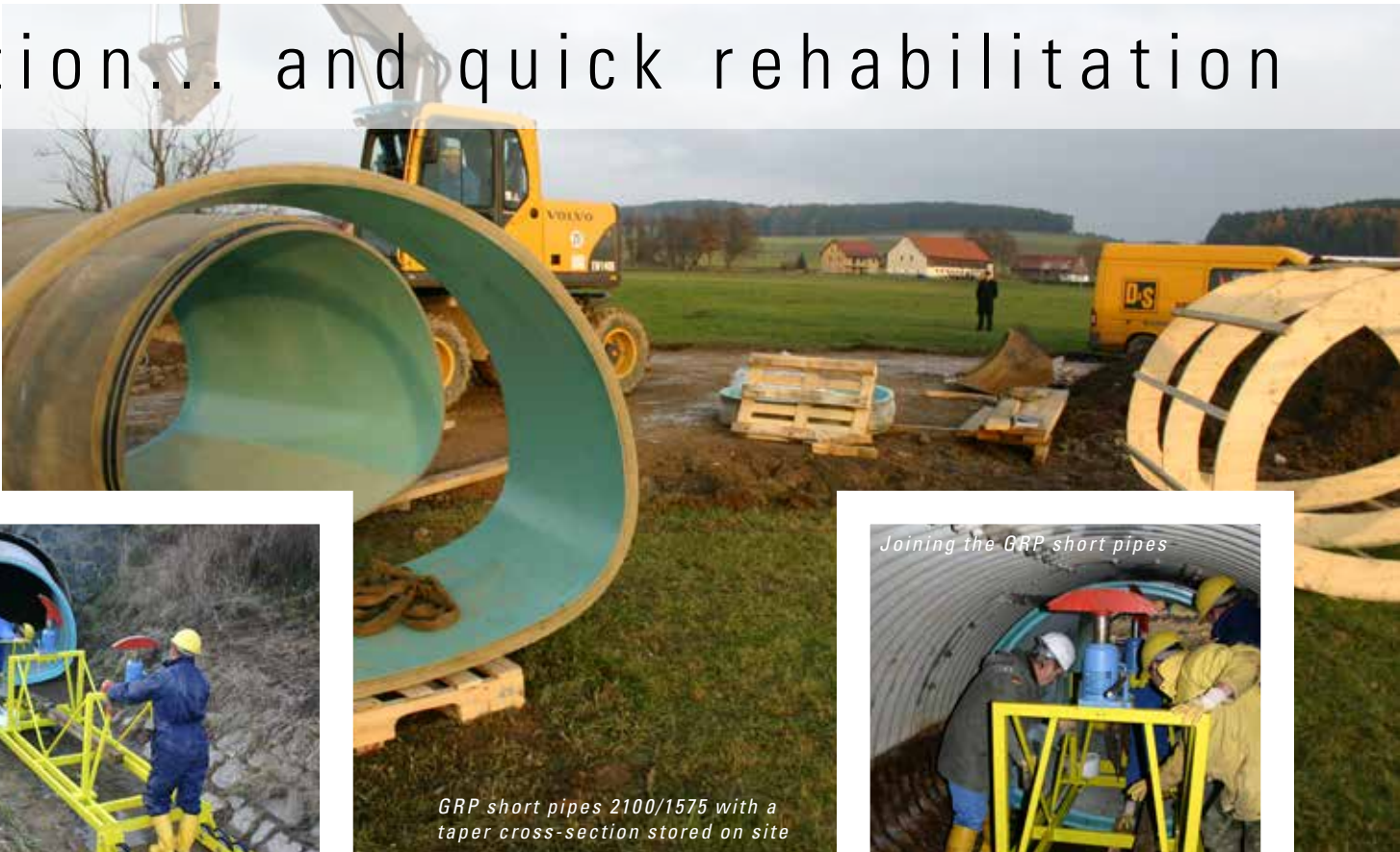
Positioning of the pipe carriage for receiving the relining section
