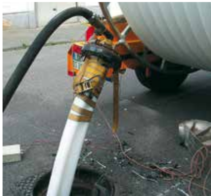
The compact pipe is inserted with the characteristic deformation
