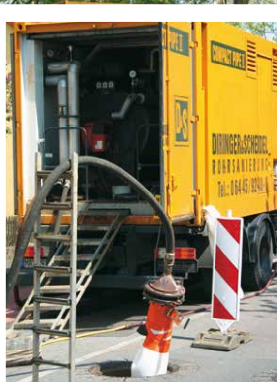
Boiler plant with steam
