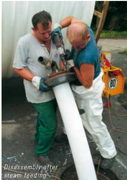
The compact pipe is inserted with the characteristic deformation
