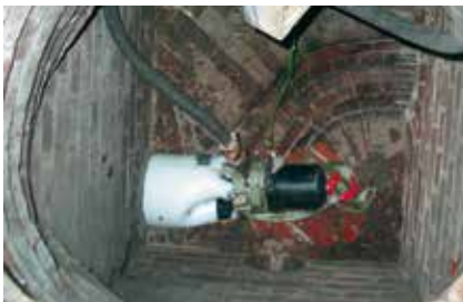
Pressure pots close the steam system
