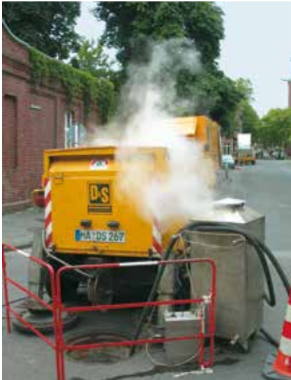
The installed compact pipe is erected with steam
